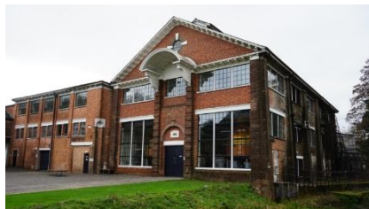
Main Still House – built in 1916 and originally housed the mill for Indian paper money.
